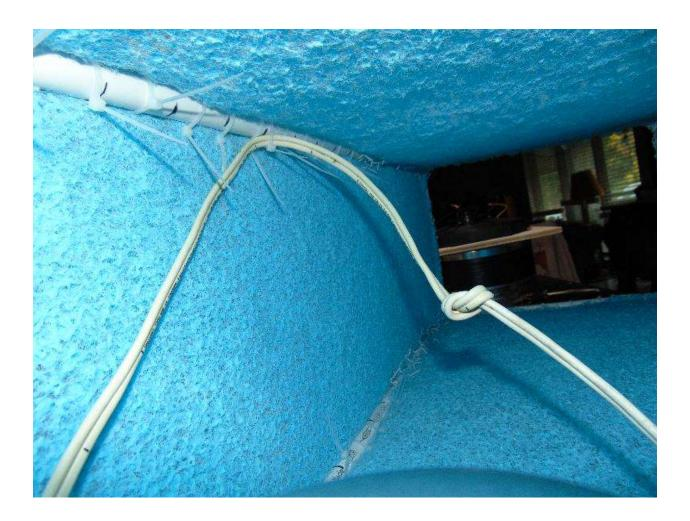
Above shows where the power cables coming into the unit are ZIP tied to the inside of the cooler about half way up inside the cooler. I pull about 3 feet more up past this ZIP tie and I tie a knot so it can not slip down.
